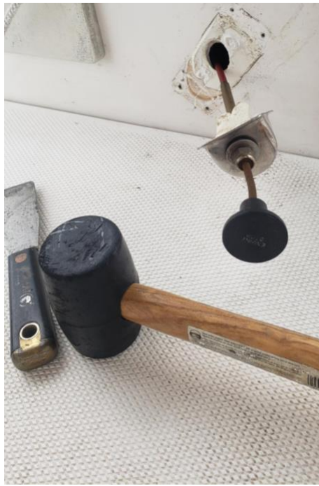
Figure 4: Stop cable pull knob at cockpit bulkhead. Note abundant rust on bent cable.
